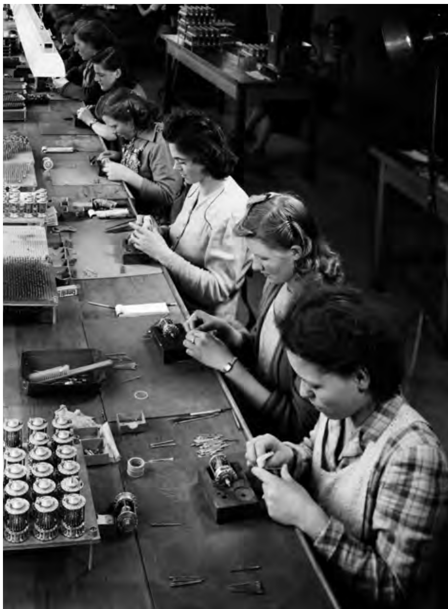
Montage Rechenmaschinen, Contina AG; v. r.: 4. Cilli Senti-Matt, 5. Waltraud Covi, 6. Irma Kaufmann-Matt, 8. Paula Meier, 1954/1955.
